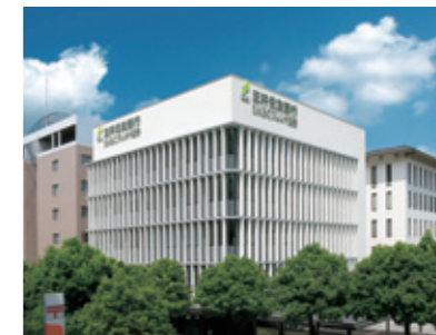
8_ 銀泉伊丹ビル Ginsen Itami Building
