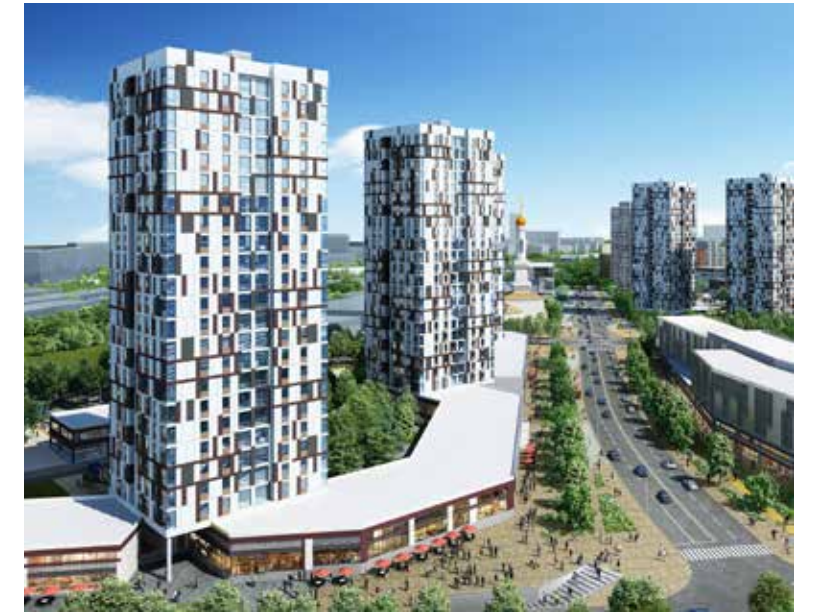
Top: Façade of the residential buildings Below: Bird's-eye view of the development
