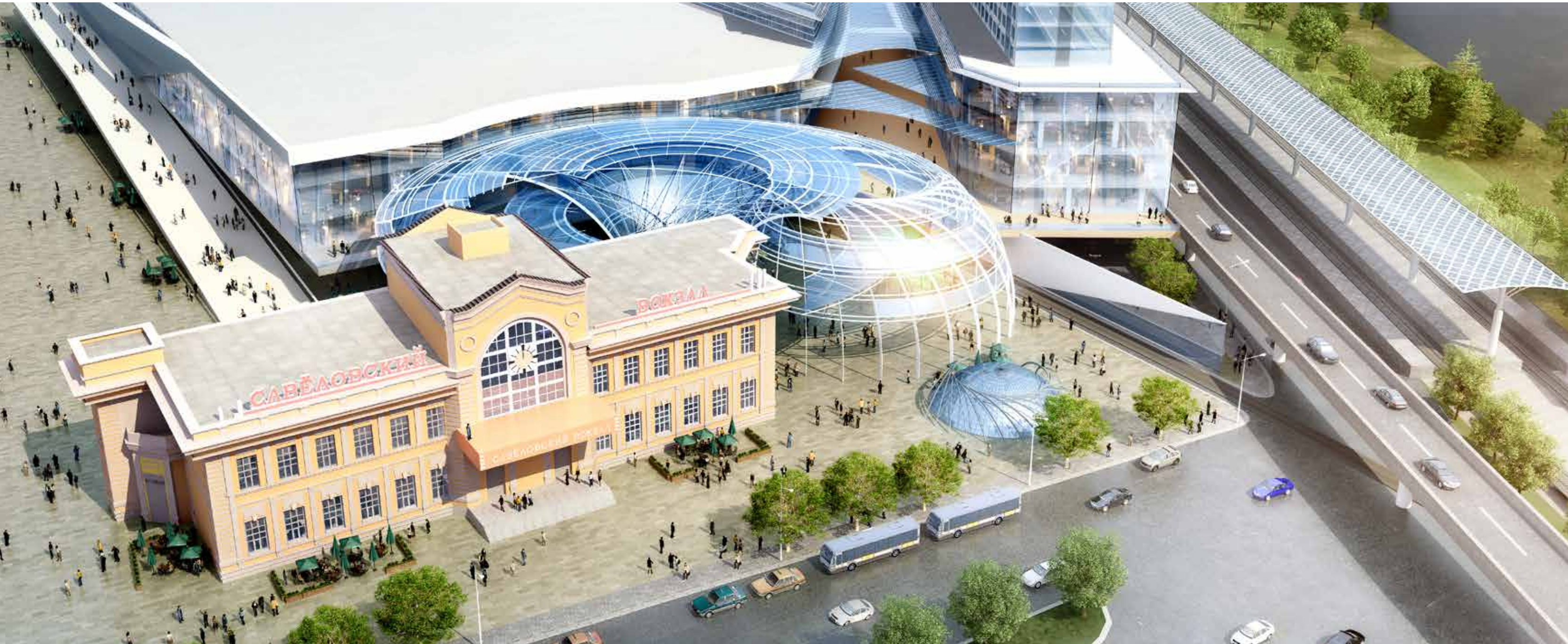
Integration of the historical station into the modern development
