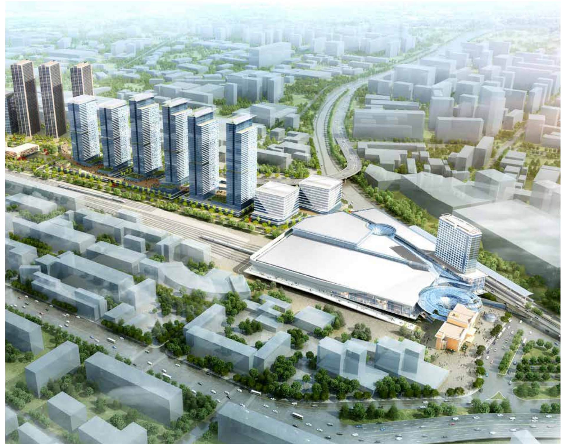
View over the Savelovskaya development
